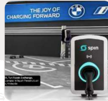
AC charger installation at BMW Malaysia
