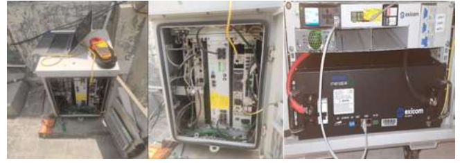
Small power solutions (<10kW) to power small cells or Wi-Fi hotspots for dense urban areas
