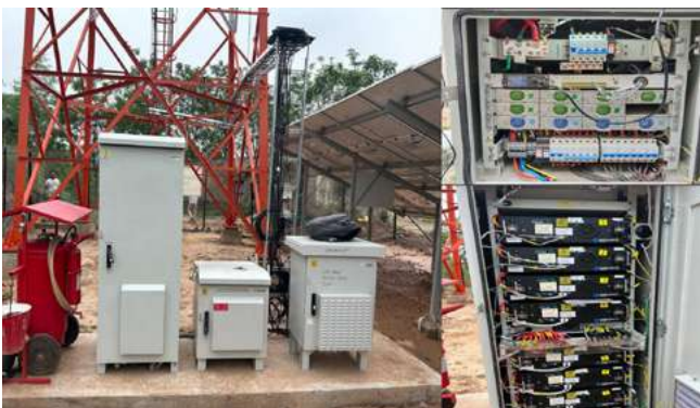
Hybrid power solutions to enable a telecom base station site powered by a combination of solar, grid and diesel genset using smart energy management
